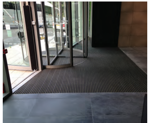
The Blade – EMS Tretford Design Range with Bronze anodised aluminium grid system
