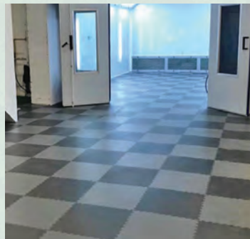
Recycled tiles are then installed in their new environment as a sustainable flooring system.
