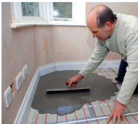
Application of smoothing compound over electrical underfloor heating system
