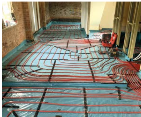
Water-based UFH system, prior to the application of smoothing underlayment and floor covering
