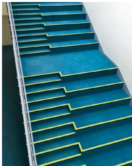
Stair nosings can help with any stair design whilst ensuring safety, Light Reflectance Values (LRVs) and minimal trip hazard guidelines are adhered to
