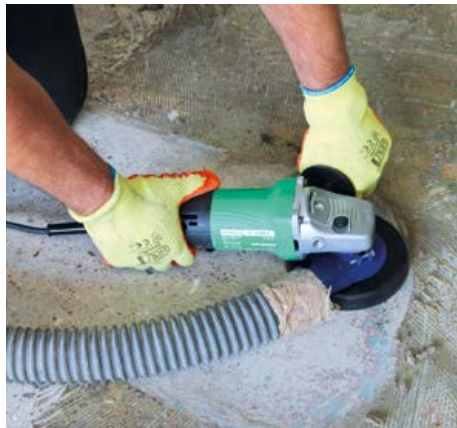
Grinding is ideal for removing paint and coatings, thin adhesives, latex and screeds, levelling compounds and elastomeric systems
