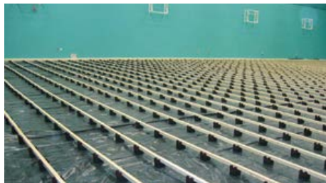
An example of a cradle and batten subfloor where the levelling capabilities of the system can be seen
