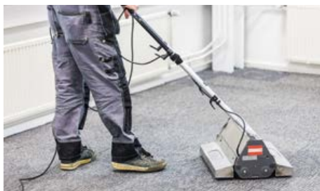
TOP AND CENTRE: Mechanical cleaning and slurry extraction being undertaken using a wet and dry rotary brush machine on textile flooring. This is a highly effective method in removing any build up of soiling; on both textile and vinyl (or soft and hard) surfaces requiring only minimal drying time before the floor is back in use.
